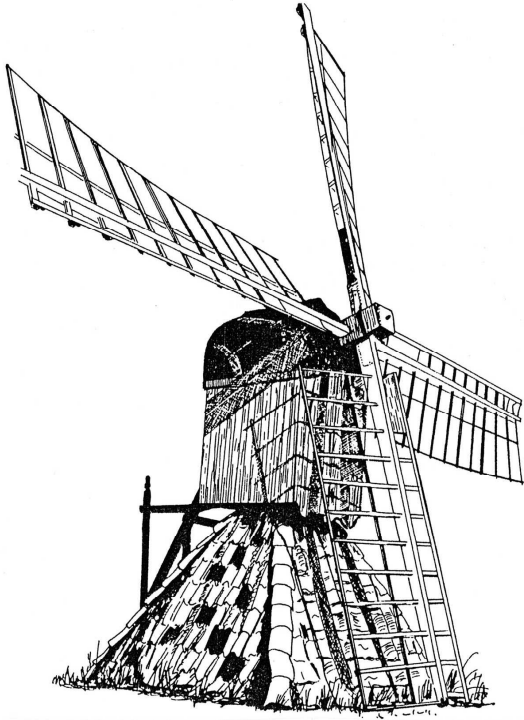
FRIESLAND SPIDER MILL with base protected by tiles.
